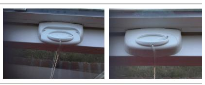
If lock on top sash hits bulb seal on the bottom sash it may need to be removed to keep the window from springing up due to compression of the lock and bulb seal when closing. May also have to slightly shave the keeper if it binds while engaging it into the lock.
