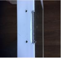
6 Reinstall bottom sash and test to make sure it works with the keepers installed.
