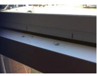
Install keepers in marked locations with #6X3/4" self tapping screws.
